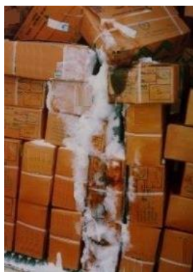
Figure 1.12 – Ice from leak in door gasket
