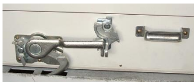
Figure 9.6 Roller shutter lock
